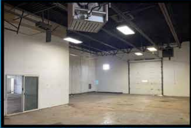
South Overhead Door
